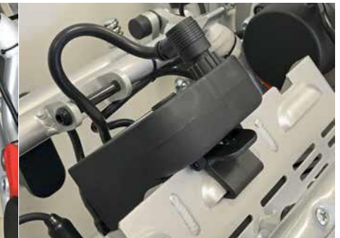
Check battery clips are secure
